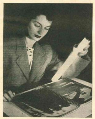
Is this the lighting of the future? The young lady's reading light consists of a fluorescent tube without wired connections. The Tesla coil that powers the tube is located in another room, but plain walls are no obstacle to its energy.
